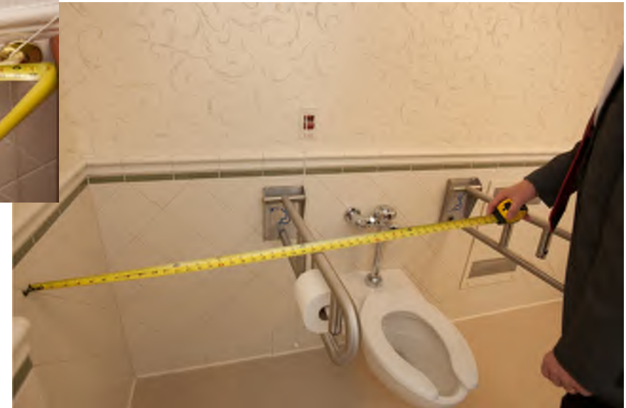
NOT ADA Compliant
